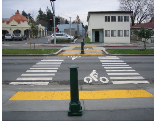
A mid-block toucan signal uses high visibility crossing markings to separate user types. (Berkeley, CA)
