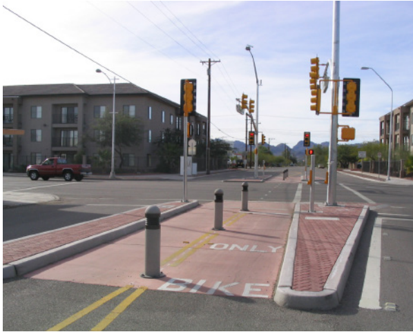
This central island also functions as a right-out channelization island for motor vehicles. (Tucson, AZ)
