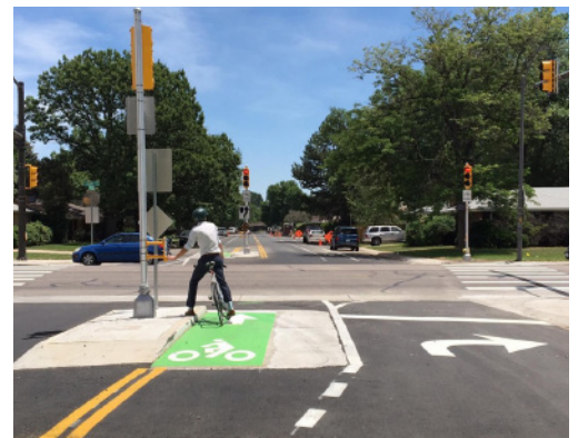
A bicycle boulevard to bike lane transition and arterial roadway Toucan crossing in Fort Collins, Colorado
